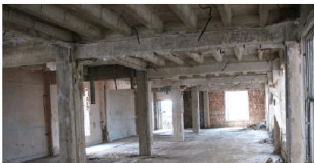
Fig. 2. Second floor of building (Looking south).
