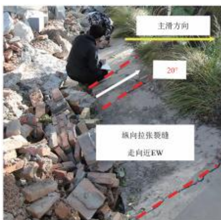
(a) 纵向拉张裂缝
